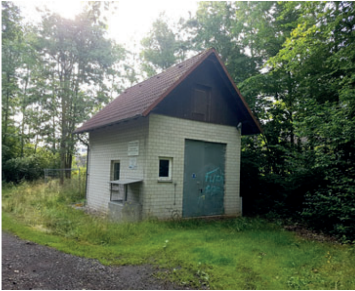
Pumpwerk Zschoner Ring
